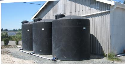
A 9,000 USG system comprised of 3 tanks that collects from 5000 sq.ft. roof supplies water for filling mobile equipment and washing equipment.
