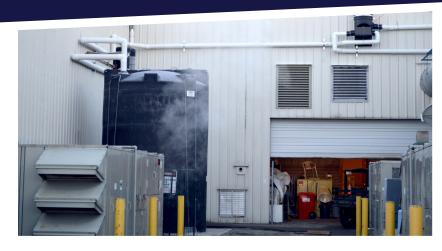
We worked with Abbotsford Water & Sewer Services to create a 8,000 USG ASTM rated poly tank system with engineered seismic tie downs. This custom rainwater system collects from 48,000 sq.ft. of roof area to collect up to 1.6 million US gallons per year to flush over 30 bathroom fixtures. It was designed to meet the demands of a tradeshow day which can commonly use up to 8000 US gallons.
