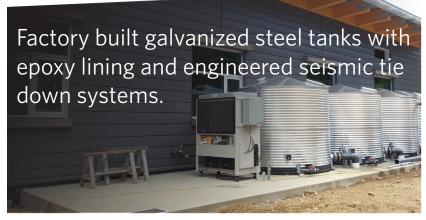
**Gabriola :** 4 – 3750 USG Galvanized steel epoxy lined tanks for toilets, vehicle wash and emergency water supply.
