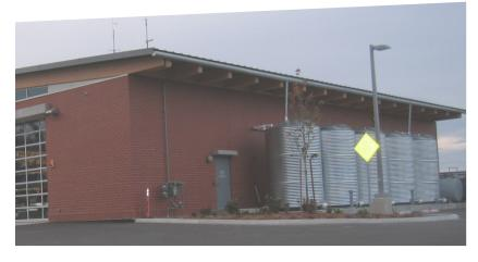
**Central Saanich:** 5 – 3718 USG Galvanized steel epoxy lined tanks for toilets, vehicle wash, tanker fill and emergency supply.
